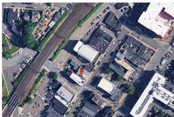
Aerial Photo of Site
